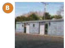
Union Hall Built: 1966, converted: 1993
