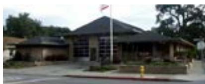
Los Gatos Fire Station #83 Built: 1964, remodeled 2002; 6,810 SF
