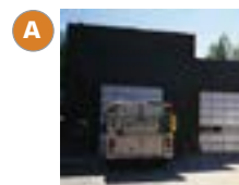
Repair Shop Built: 1980, remodeled 2009
