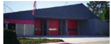
Seven Springs Fire Station #72 Built: 1992, remodeled 2003; 9,120 SF
