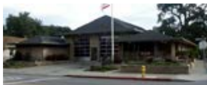
Los Gatos Fire Station #83 Built: 1964, remodeled 2002; 6,810 SF
