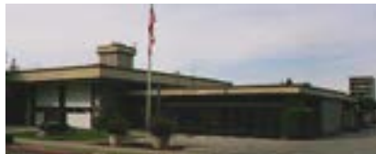
Sunnyoaks Fire Station #80 Built: 1969; 6,040 SF
