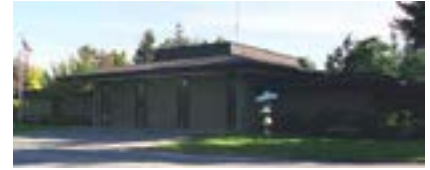
Los Altos Fire Station #75 Built: 1968, remodeled 2002; 9,350 SF
