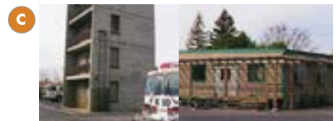
McCormack Training Center Drill Tower Built: 1969 Classrooms Built: 1996
