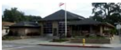
Los Gatos Fire Station #83 Built: 1964, remodeled 2002; 6,810 SF
