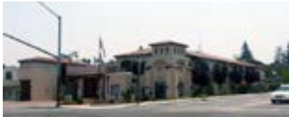
Saratoga Fire Station #73 Built: 1923, rebuilt 2004; 15,435 SF
