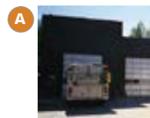
Repair Shop Built: 1980, remodeled 2009
