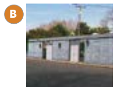
Union Hall Built: 1966, converted: 1993
