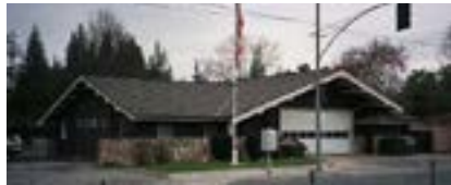
Loyola Fire Station #76 Built: 1953, rebuilt: 1998; 2,400 SF
