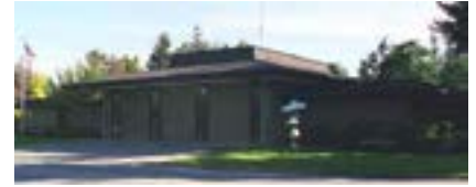
Los Altos Fire Station #75 Built: 1968, remodeled 2002; 9,350 SF
