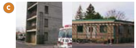
McCormack Training Center Drill Tower Built: 1969 Classrooms Built: 1996
