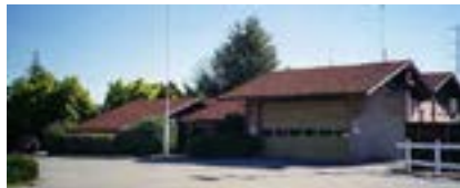
West Valley Fire Station #79 Built: 1965, Remodeled: 2003; 3,140 SF
