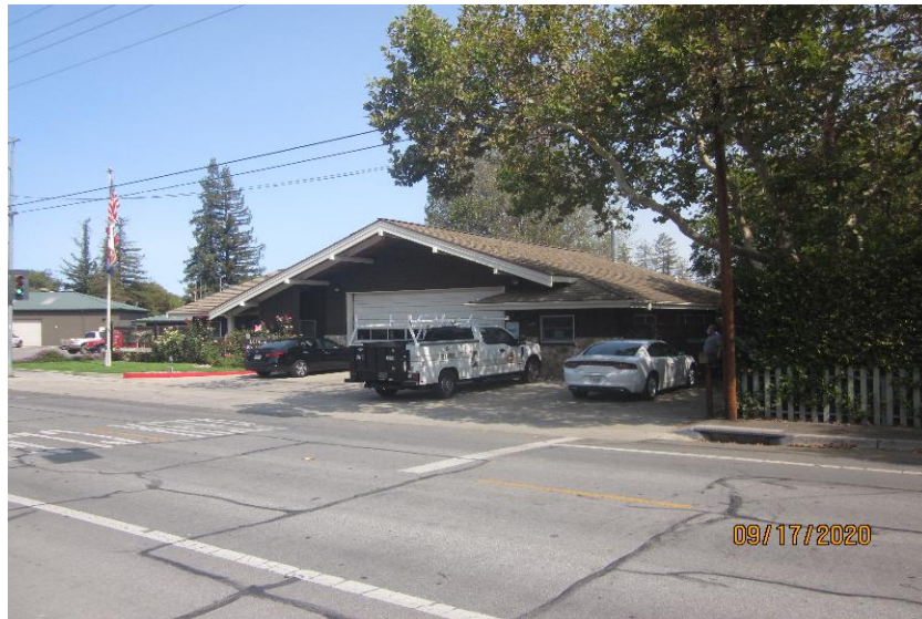
Loyola Fire Station - Site
