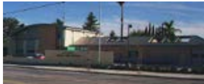
Monta Vista Fire Station #77 Built: 1966, Replaced 1997-1998; 7,100 SF
