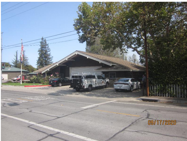
Loyola Fire Station - Site
