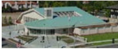
Cupertino Fire Station #71 Built: 1948, remodeled 2001; 12,775 SF
