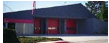
Seven Springs Fire Station #72 Built: 1992, remodeled 2003; 9,120 SF
