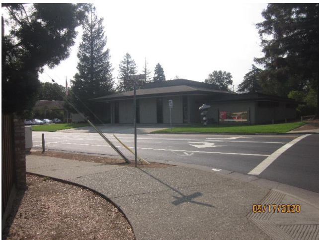
Los Altos Fire Station - Site
