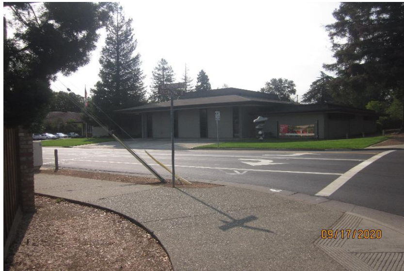
Los Altos Fire Station - Site
