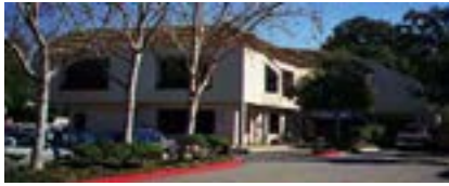
Headquarters (HQ) Built: 1984; 19,030 SF
