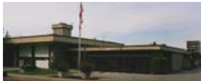
Sunnyoaks Fire Station #80 Built: 1969; 6,040 SF
