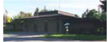
Los Altos Fire Station #75 Built: 1968, remodeled 2002; 9,350 SF
