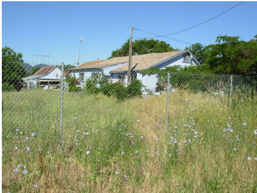
Photo 6: Single family residence on the site, looking south from Monterey Road
