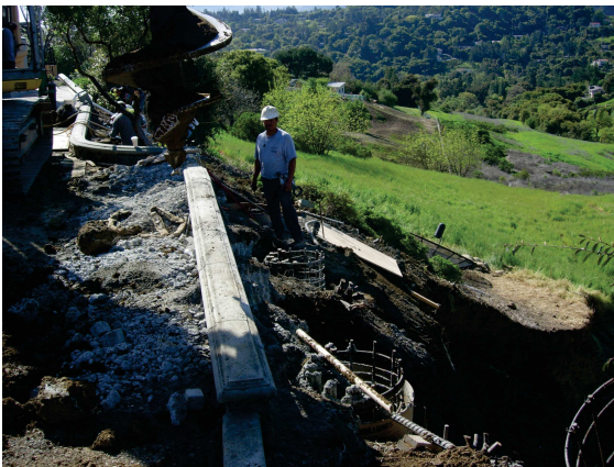
Example of a Stitch Pier Wall under construction
